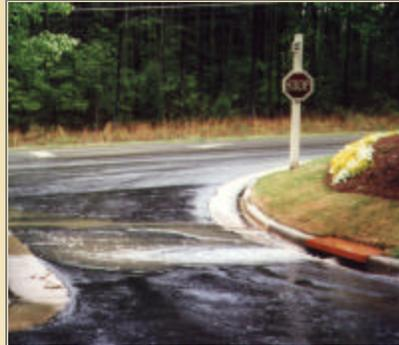
**Install a gravel drive to help keep sediment on the site and prevent it from being tracked onto the road.**
