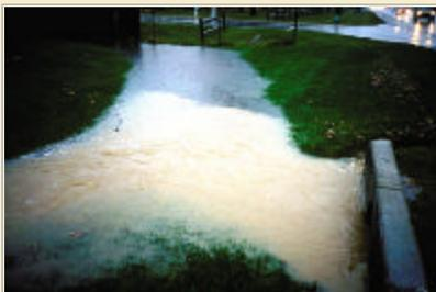
**Sediment in roads caused by construction site runoff can be a safety hazard.**
